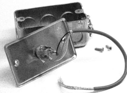
The splice point should stay inside of each junction box. That is, you want to feed the long run of cable into the box rather than
